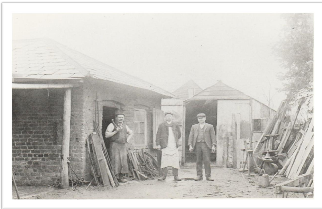
THE WHEELWRIGHT'S AND BLACKSMITH'S SHOP EARLY 1900S
